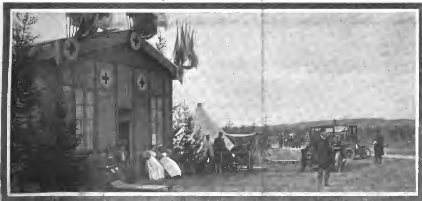
At the Rheims Tournament the Hospital Service and Emergency Equipment Was Complete in Minutest Detail
